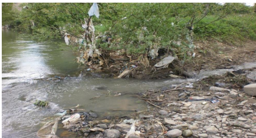
Figure 9 Sewer outlet of Bošnjanska Mahal 4.
